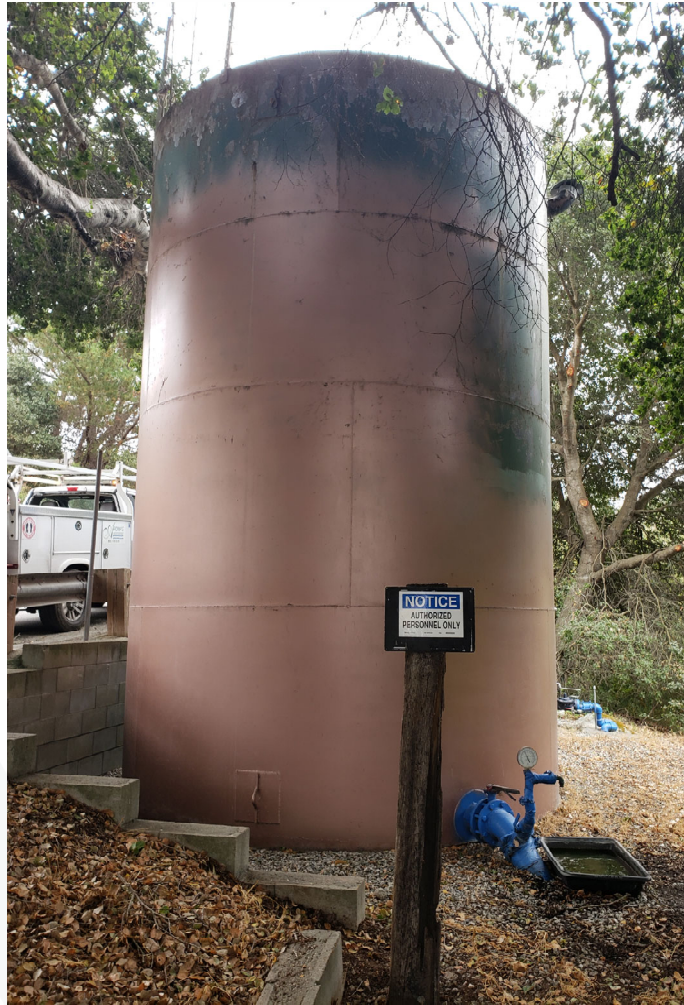
Figure 1: Existing School Road Tanks
